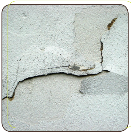
Cracked plaster wall
